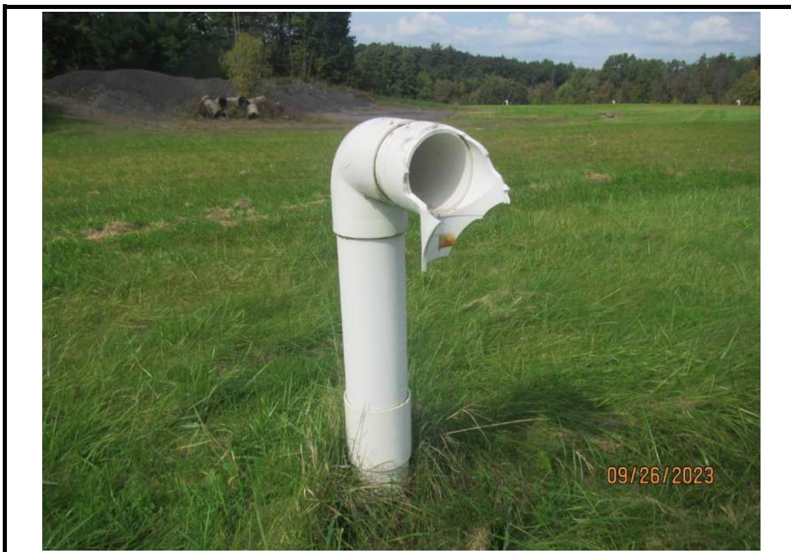
Photo #11 (facing northwest): View of damaged landfill gas vent in southern portion of landfill cap.
